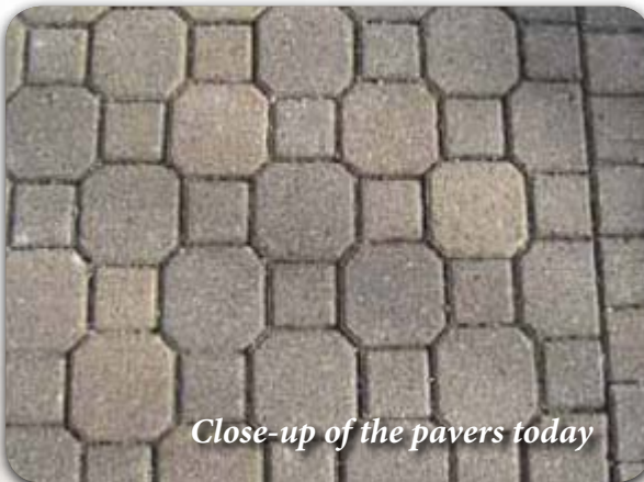
Bob Steffes installed this Borgert walkway 30 years ago
